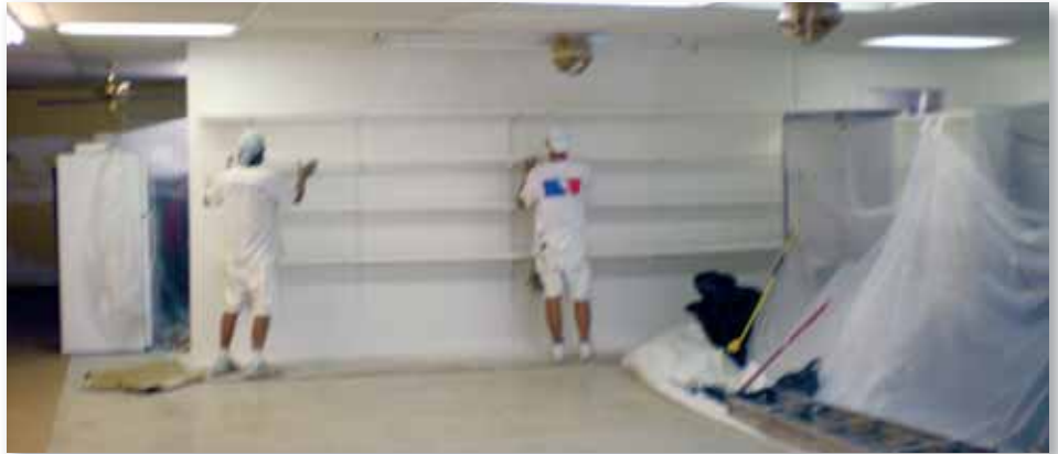
Remodeling in progress, walls are down and shelves being installed.
